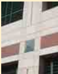
Fig. 1: Light and deep sandblast with granite and terra-cotta inserts.
