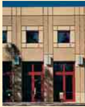
Fig. 3: Retarded and acid-etched finishes.
