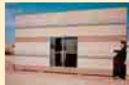
Fig. 7: Multiple mixes with acid-etched finish.
