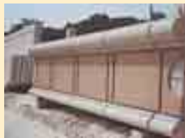
Fig. 6: Multiple mixes with sandblasted and acid-etched finishes.
