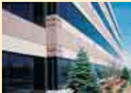
Fig. 5: Multiple mixes with acid-etched and form-liner finishes.
