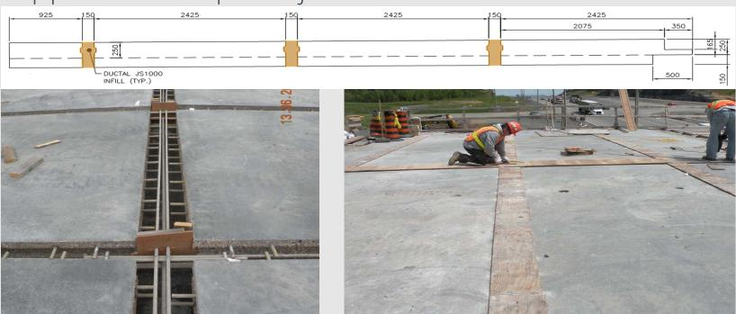
Sidewalk/parapet wall panel joints
