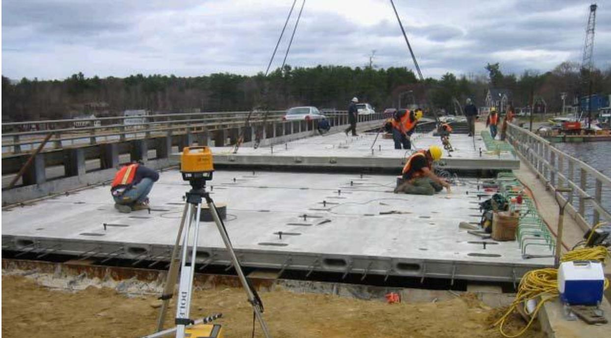
Figure 12: Placing precast deck slabs. (Source: PCI)
