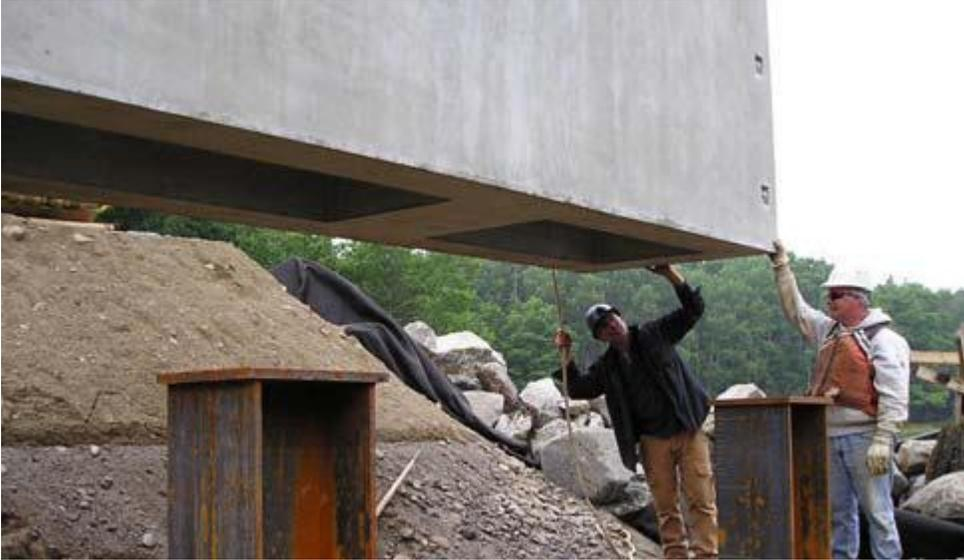
Figure 6: Placement of precast abutment section. (Source: PCI)
