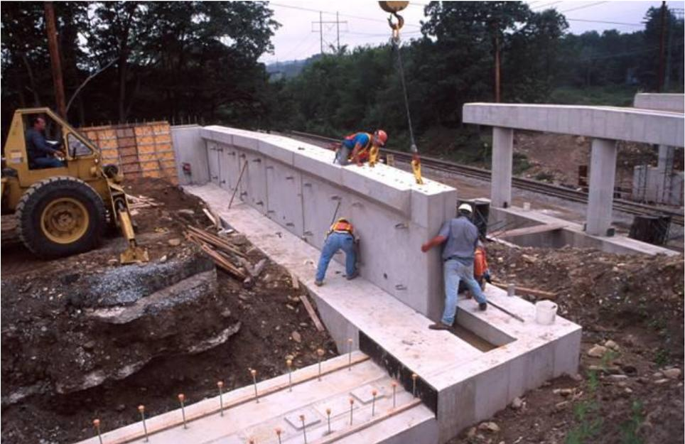
Figure 7: Precast abutment with pin connection. (Source: PCI)
