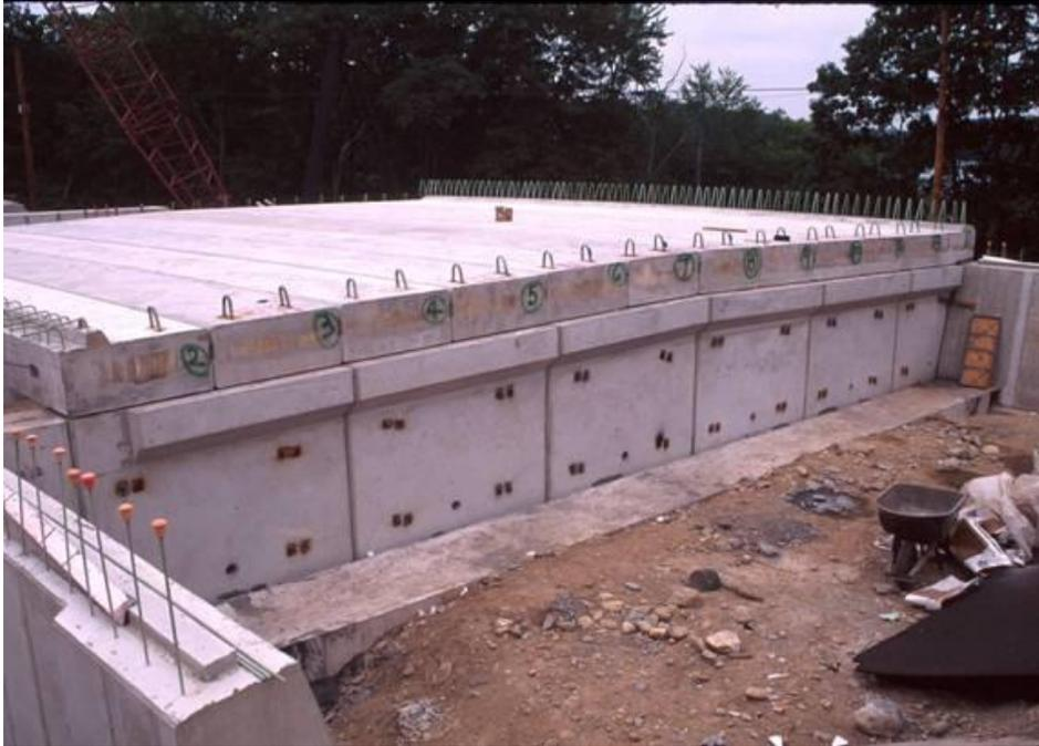
Figure 10: Completed integral precast abutment section. (Source: PCI)
