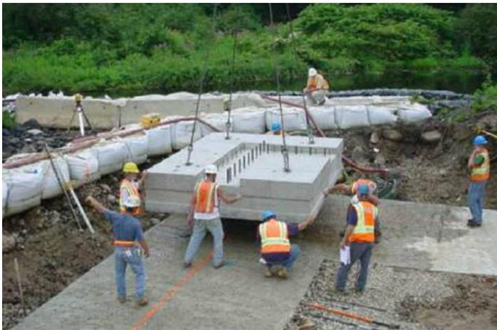
Figure 3: Placing the precast footing on the sub-footing. The sub-footing does not need to be formed. (Source: PCI)
