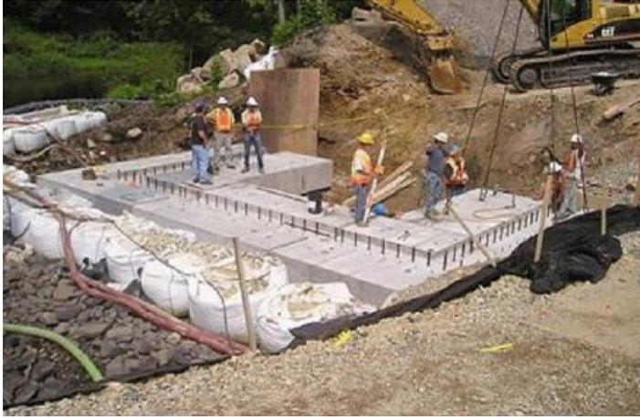
Figure 4: Completed segmental precast footing. (Source: PCI)
