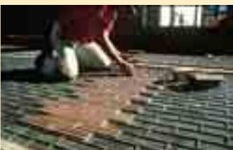
*Fig. 8: Thin brick is shown being placed in an elastomeric form liner.*
