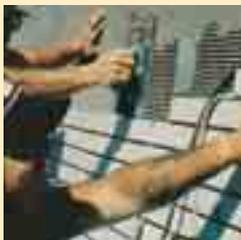
Fig. 10: Glazed thin bricks are tapped into mortar using a rubber mallet.
